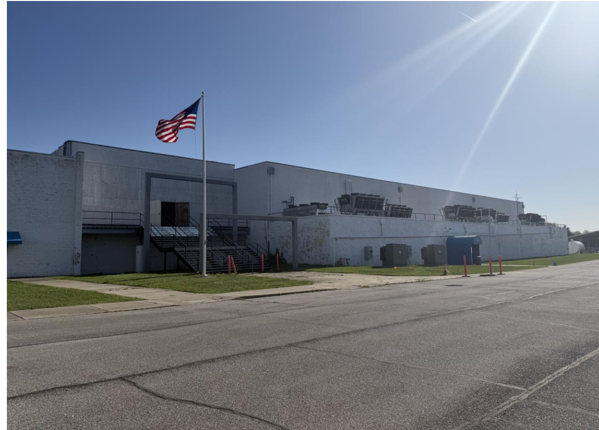
East Gate Datacenter in Indianapolis, IN
