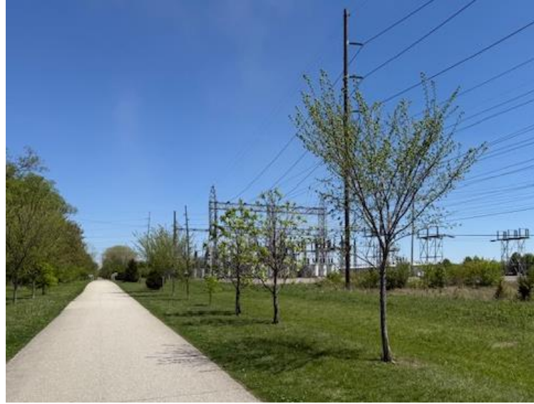
Facing East at Substation
